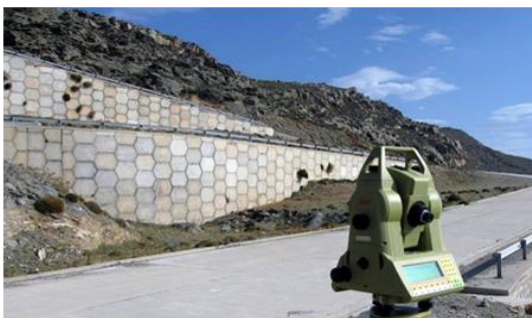
Automatic surveying system (ATS)
